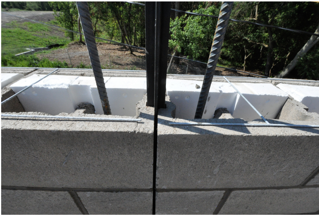
Building a control joint with a 12" Hi-R H Jamb
