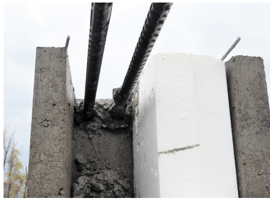
Building a bond beam with a 12" Hi-R H
