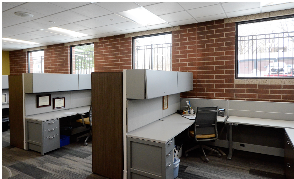
Photo below shows that same area on the interior.
