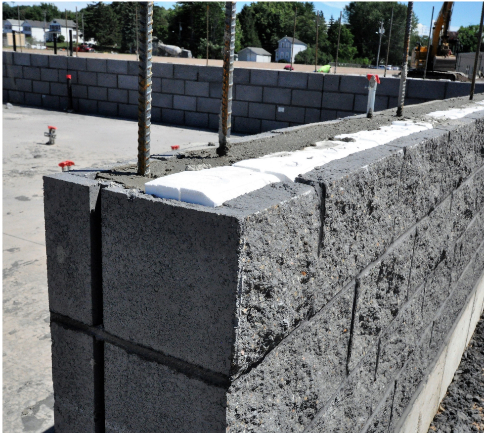
Building a door opening with a 12" Hi-R H Jamb CMU
