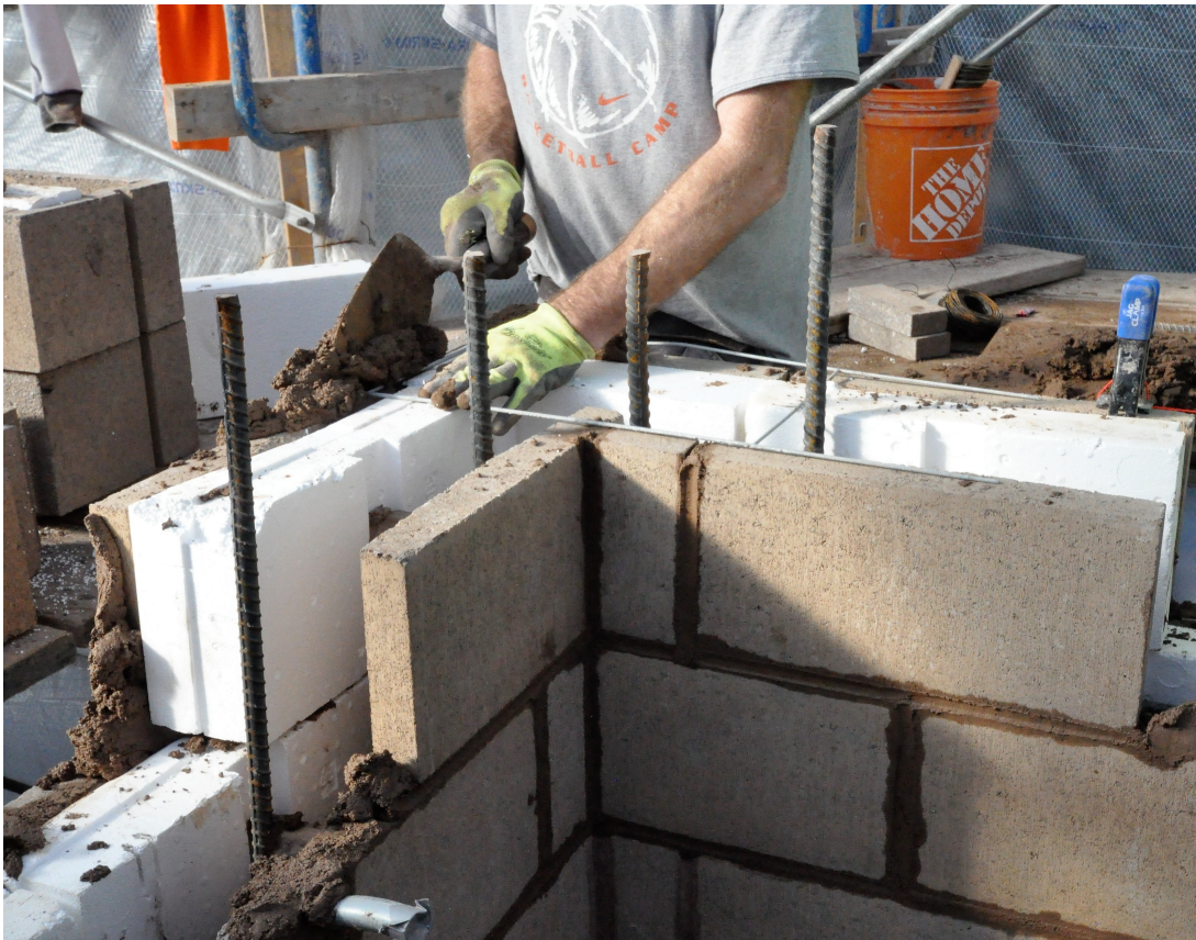
Building a corner with 12" Hi-R H L-Shape Corner
