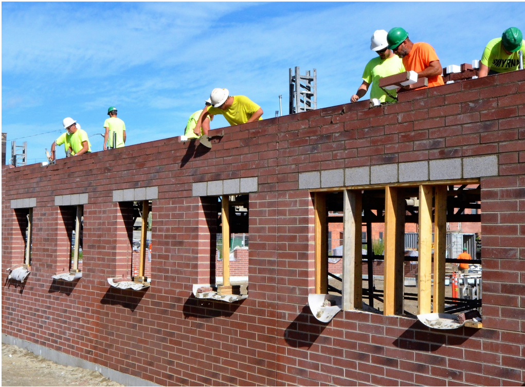
Photo above shows exterior Spec-Brik Hi-R H being constructed
