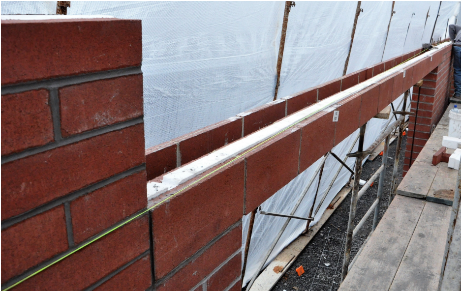
Building a lintel with 12" Hi-R H Lintel units.
