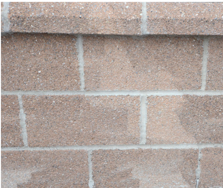
Both of these walls have been damaged cleaning with a water pressure washer that was too aggressive
