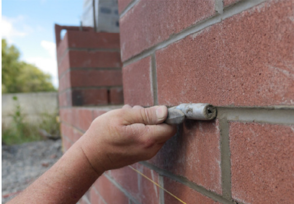
Mortar is thumbprint hard when the image of your thumbprint can be left in the mortar
